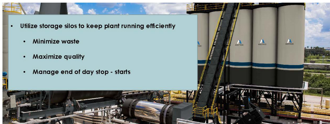
FIGURE 17 Efficient plant operation: What can be done now?
